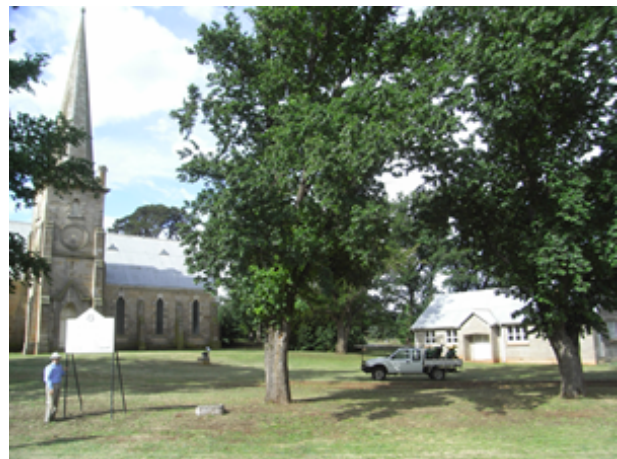
1857 Church & 1955 Hall DPIPWE, 2011
