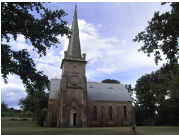
Former St Andrew's Church, 1857 Church DPIPWE, 2011
